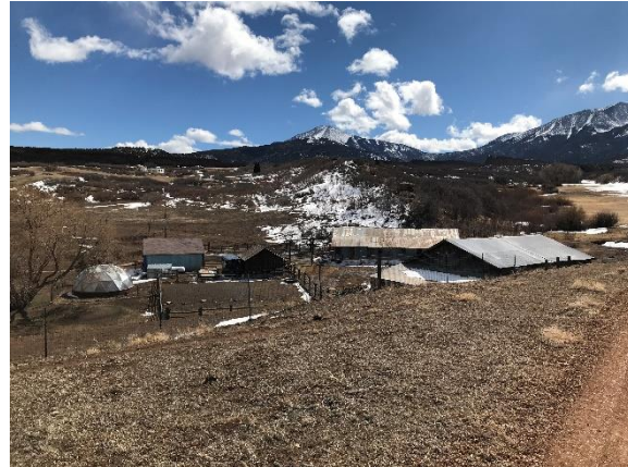
Picture 5: Older building materials are present on some structures.
