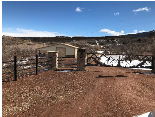
Picture 2: Hardened structure with updated building materials and improved defensible space.
